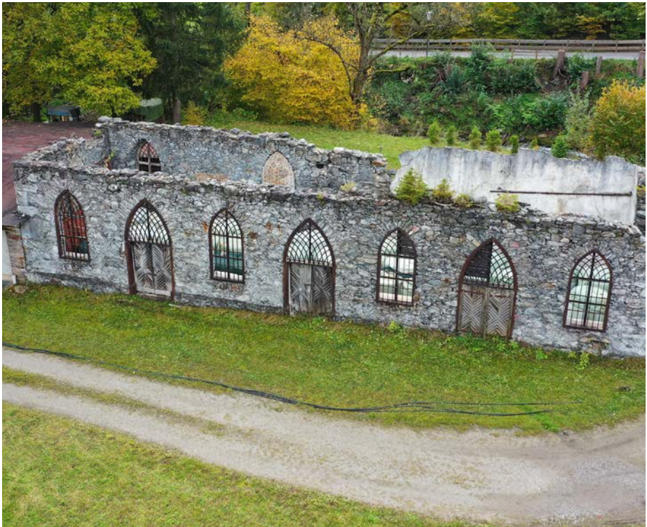
The hammer mill at Fügen processed local iron ore until the 20th century (photo F. Messner)
