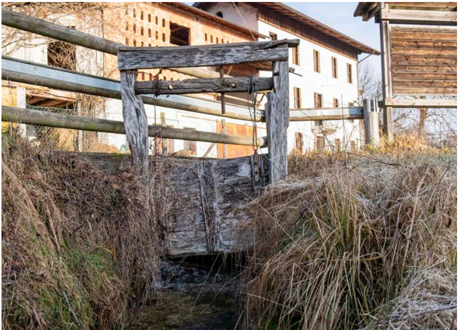
Sluice gate for diverting the flow from the channel near the former Bugana sawmill (photo T. Meneguz)
